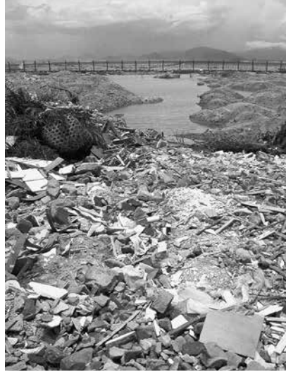
Fig. 7: Reclamation site on the northeastern banks of the Nantou Peninsula, 2003. Significantly, 20 years into urban construction, both earth (from local mountains) and architectural debris (from first-generation buildings) were used to »fill the sea.« In the middle ground are fishing nets and, in the background, the Yuen Long mountains, Hong Kong New Territories.
